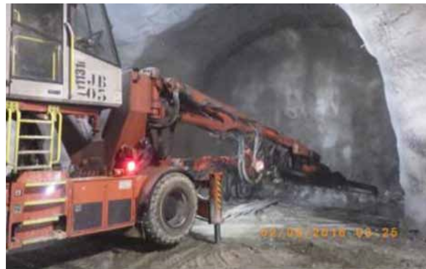
Saint-Martin-la-Porte Niche PM 1450- Foration du front
